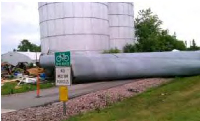
Figure 3.98. Severe Thunderstorm Caused Grain Bin Collapse, July 11, 2011
