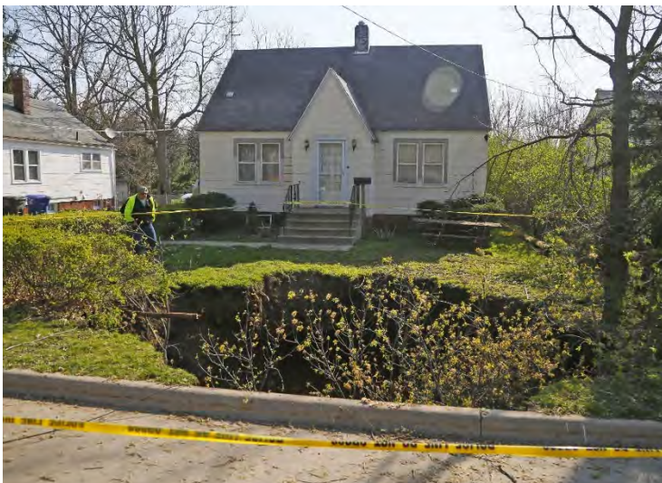
Figure 3.93.2: April 13, 2016 40-foot sinkhole opened up in south side Des Moines front yard. Source: Des Moines Register
