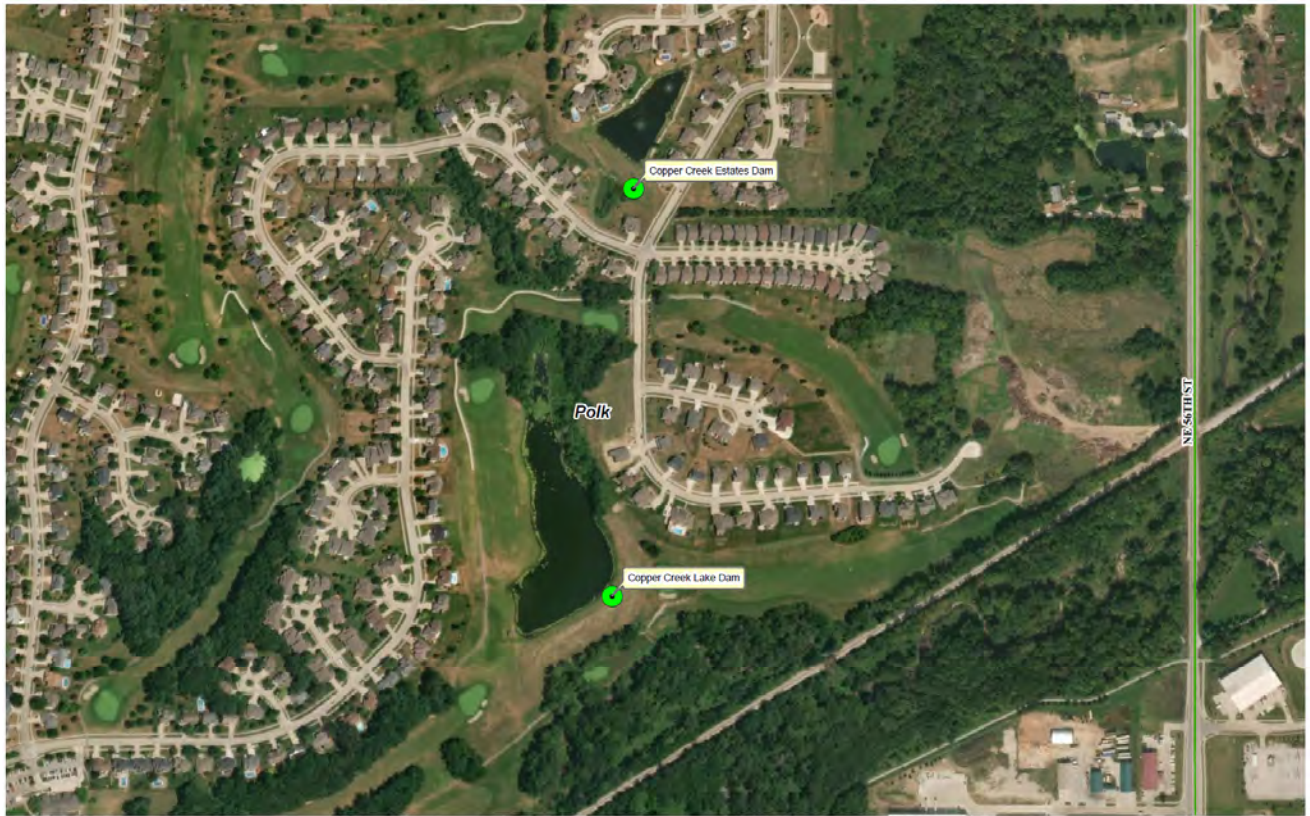
Figure 3.40. Copper Creek Estates Dam and Copper Creek Lake Dam
