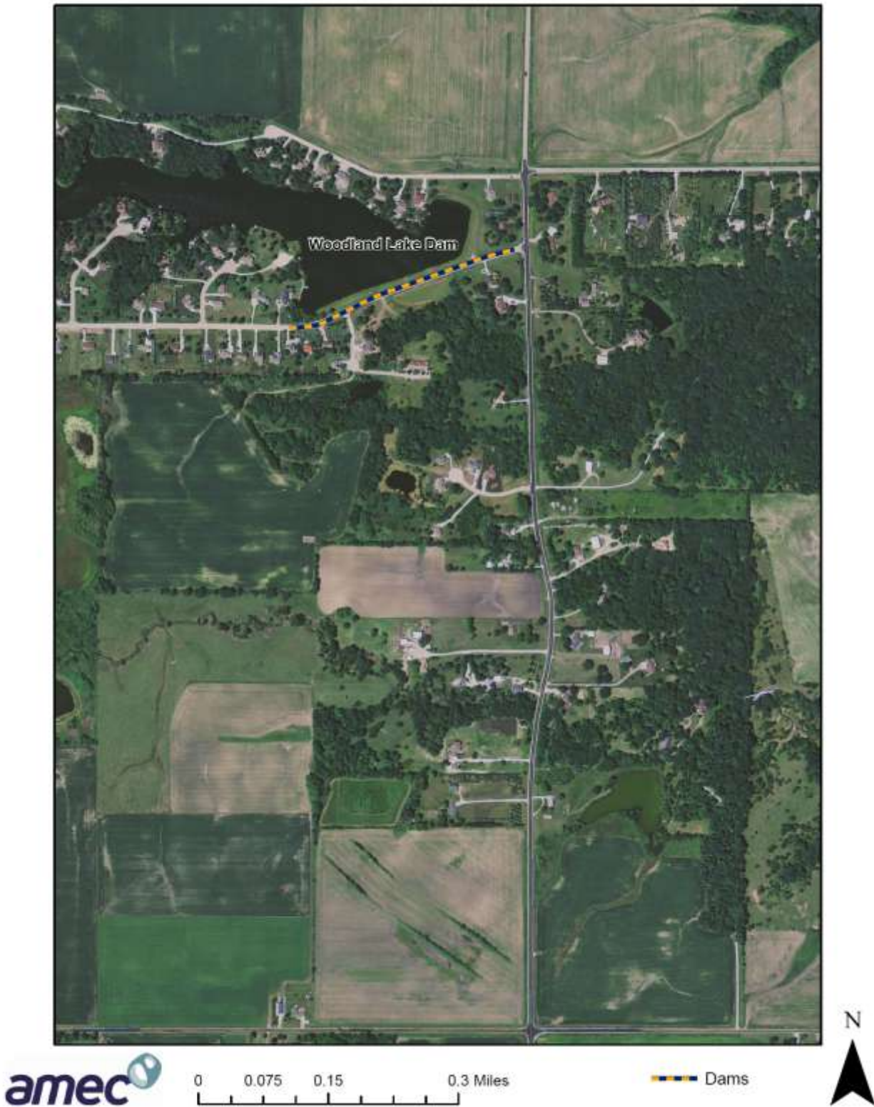
Figure 3.45. Woodland Lake Dam
