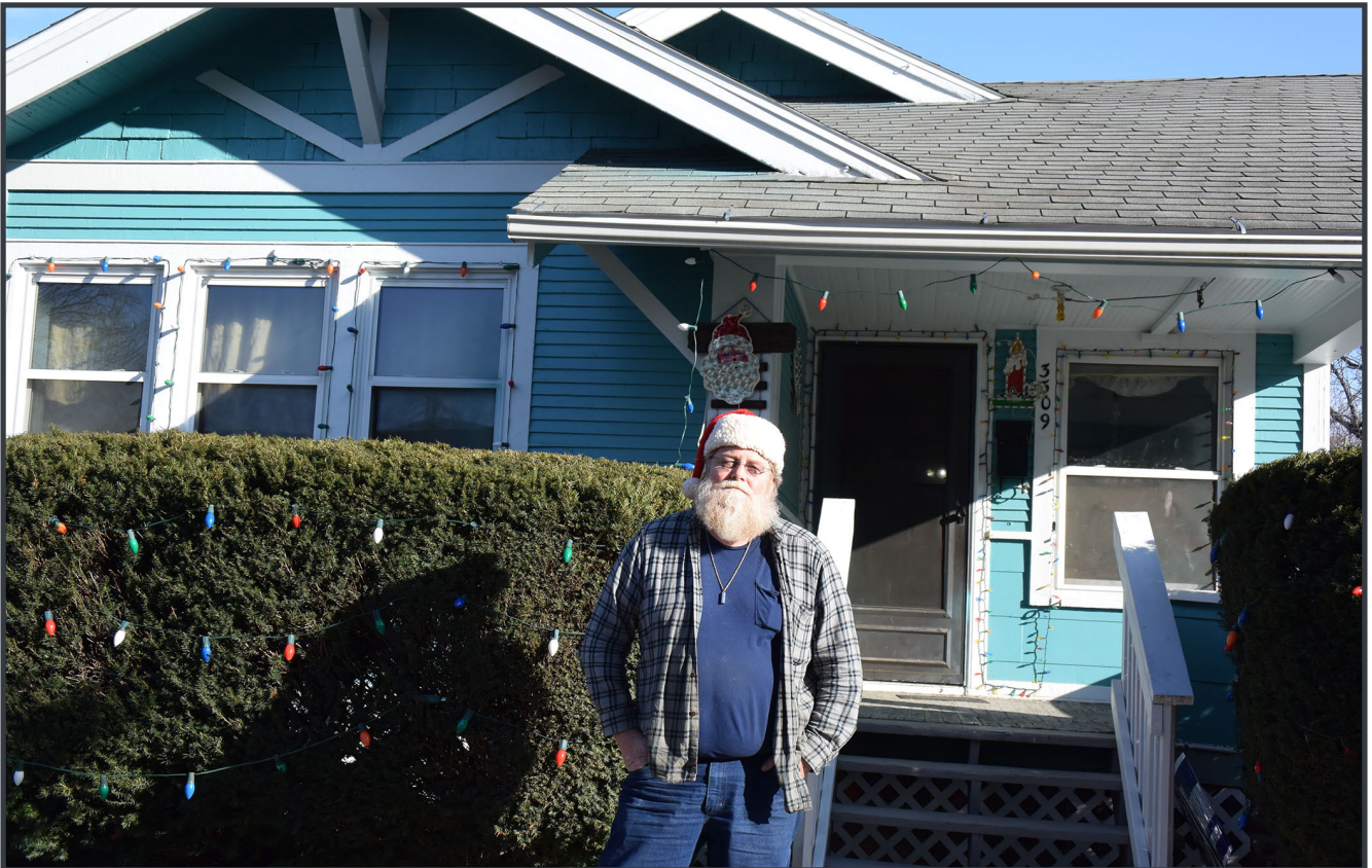
Jack L. Corbin in front on his newly remediated lead safe home.
