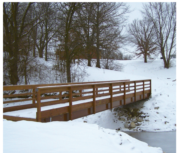
Improved bridge over the newly acquired and enhanced Oakview Pond at Yellow Banks Park.
