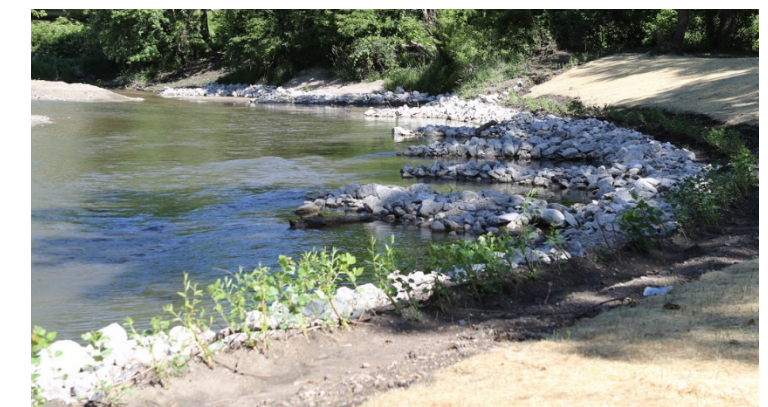
2. Recently completed stream restoration
