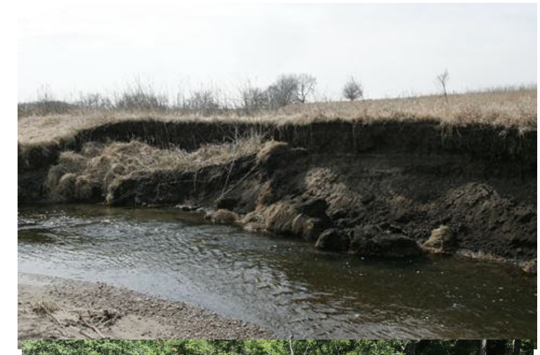
1. Example of streambank erosion
