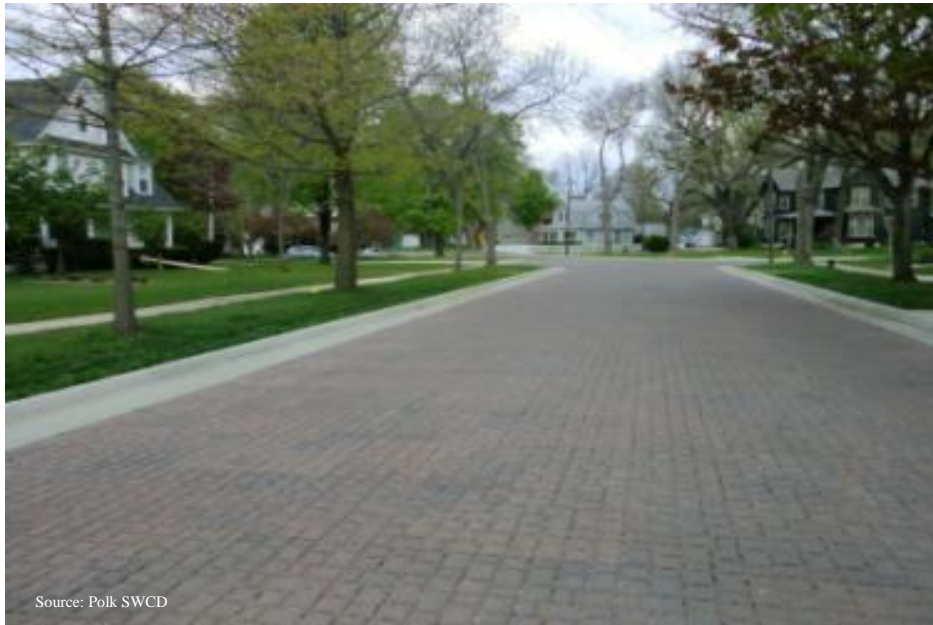
Figure 6-7: Permeable Pavers
