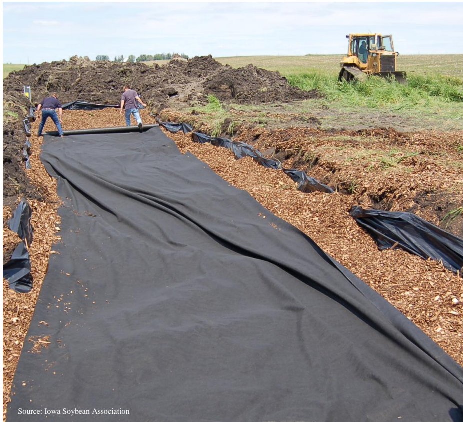
Figure 6-12: Bioreactor Being Installed in a Field
