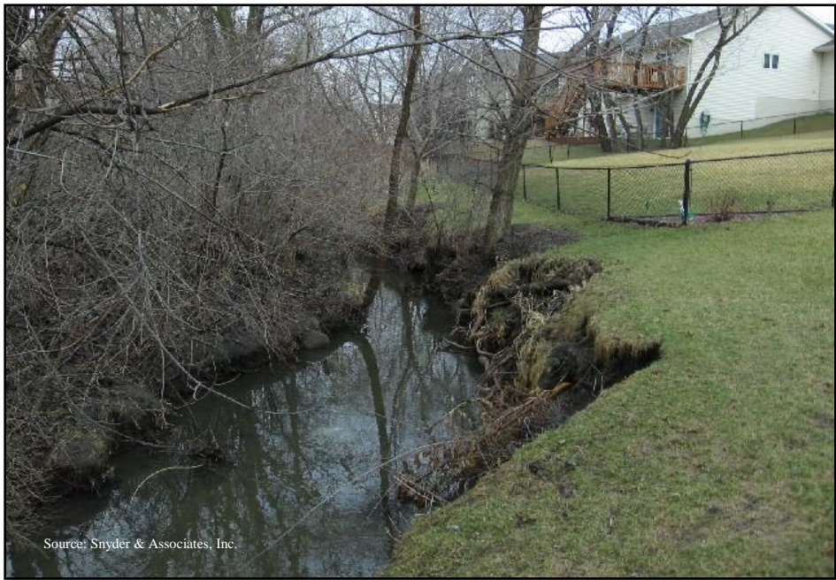
Figure 6-3: Eroding Bank before Stream Restoration
